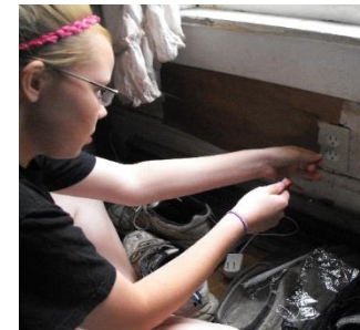
Stephanie is installing a draft stopper to help stop cold air from entering the home
